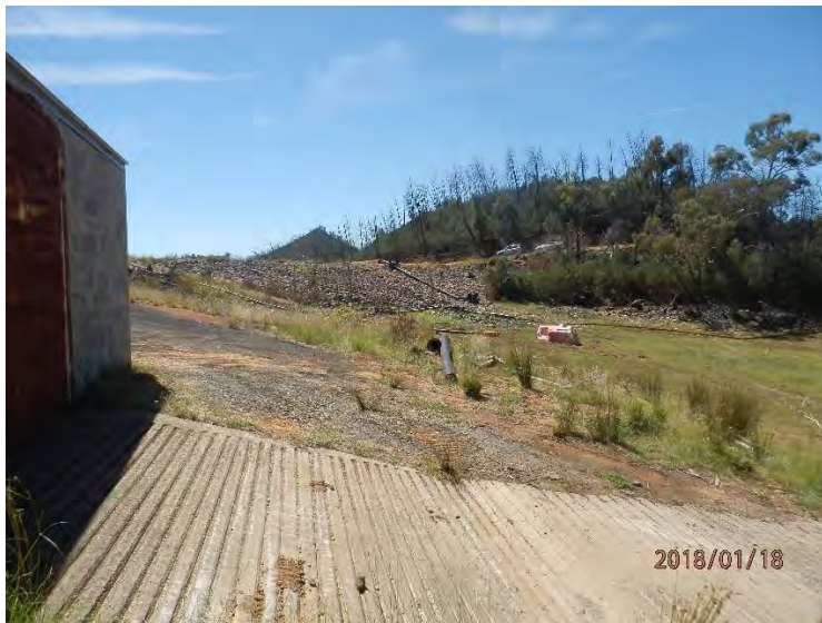
Photo 7-1: Access between existing boat shed and saddle dam
